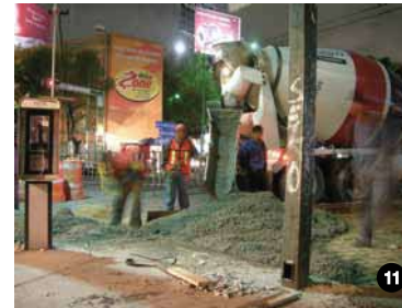
Intersection during construction period
